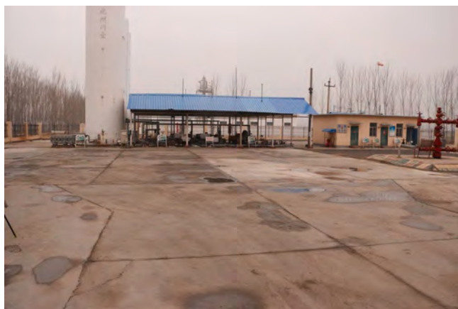
Fig. 3. Sinopec Gao-89 Block CO 2 injection facility. (Photo: Ning Wei, 2014).
